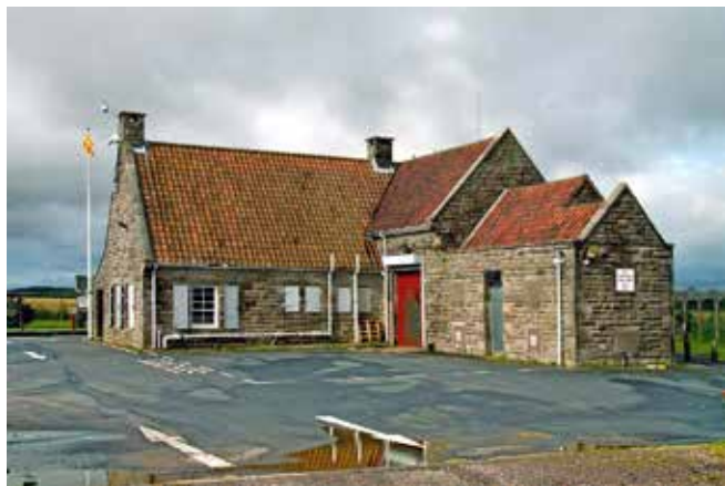
The Anstruther guard house was built of local stone to blend in with other buildings in the locality. Photo Dave Cleghorn
